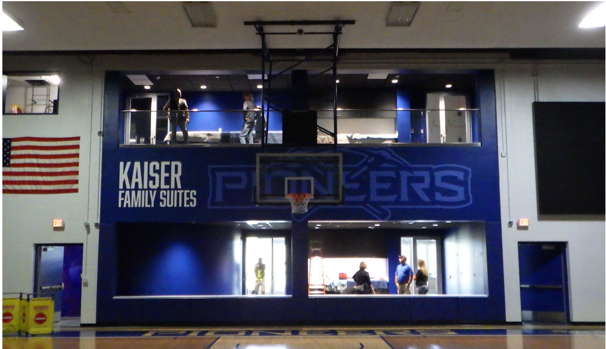
UW-Platteville, Williams Fieldhouse Seating Renovation Project budget: $800k. Substantial Completion: September 2024
