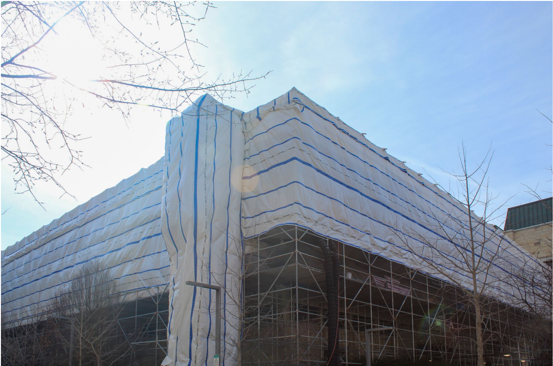
UW-Madison, Elvehjem Building Envelope Renovation Project budget: $12.1M. Substantial Completion: July 2025
