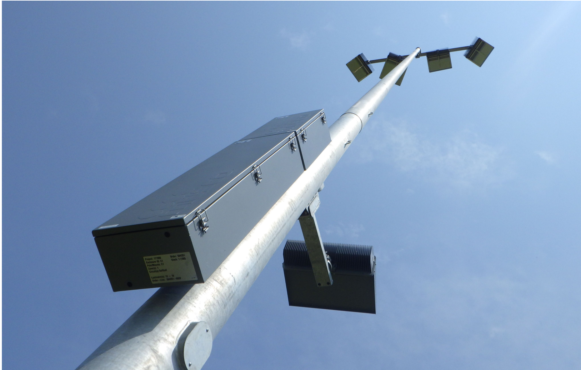
UW-Whitewater, Softball Field Lighting Project budget: $300k. Substantial Completion: August 2024
