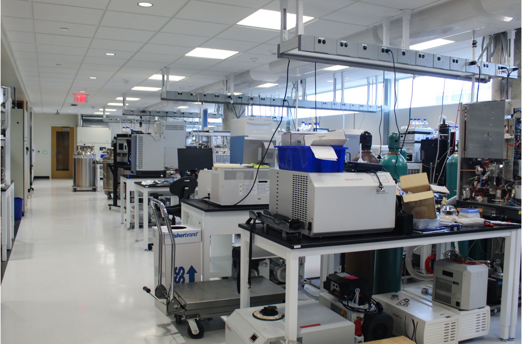
UW-Madison, DeLuca Biochemical Coon Lab Renovation Project budget: $2.3M. Substantial Completion: August 2023
