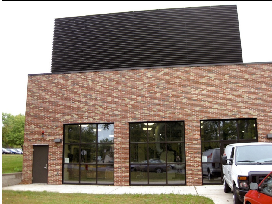
Chilling Plant - Exterior
