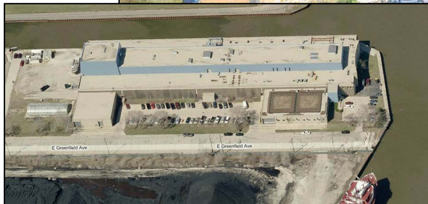
Great Lakes Research Facility (GLRF) - Before
