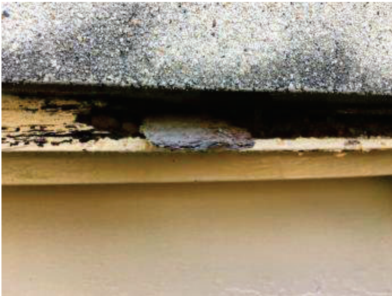
Photos 10,11. Examples of rusted and rotated steel angle lintels
