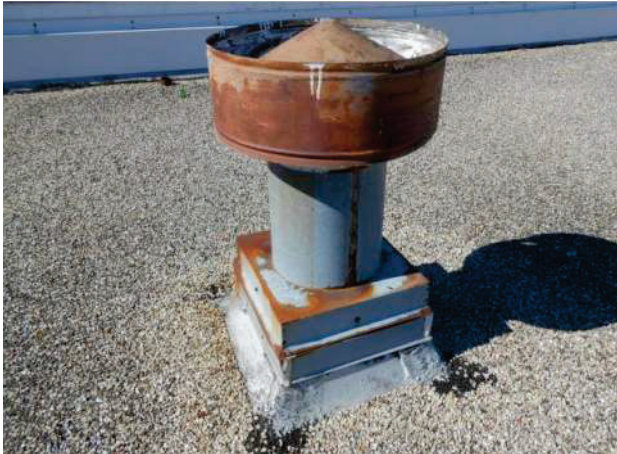
Photo 23. Example of flashing surrounding the curb
