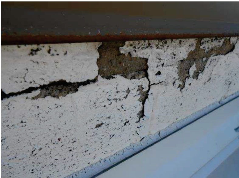
Photo 17. Inner parapet surface construction
