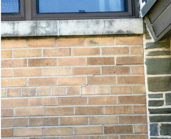
Photos 2-3. Stepped cracks in the exterior brick façade
