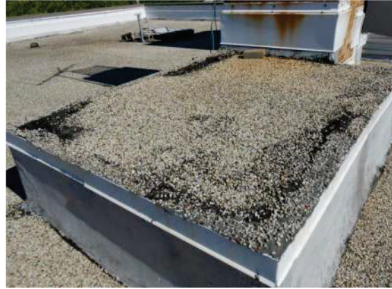
Photo 15. Example of bare spots and patching
