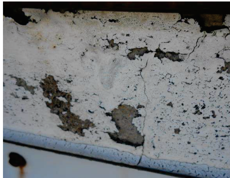
Photo 20. Example of line sealant and spalling surface
