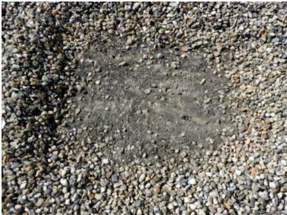
Photo 16. Example of bare spots and patching
