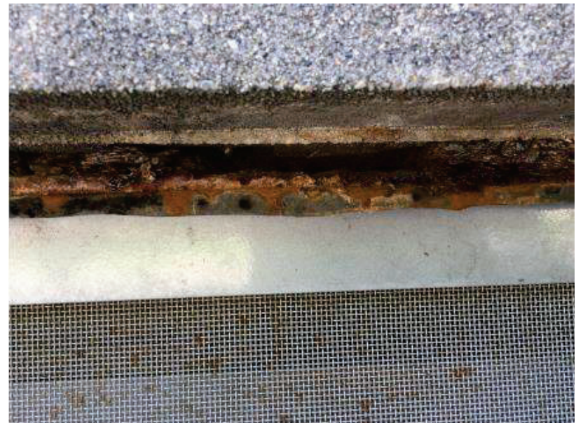
Photos 10,11. Examples of rusted and rotated steel angle lintels
