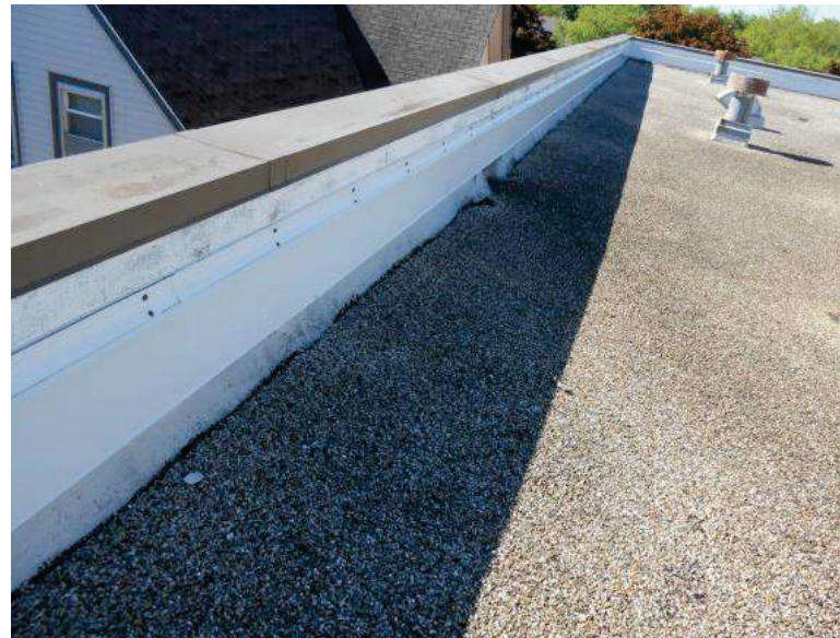
Photo 18. Wall steel coping
