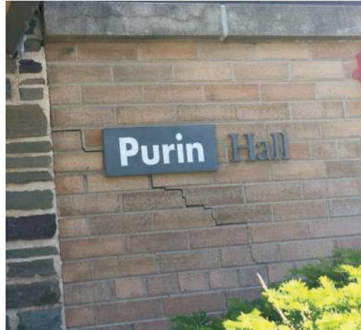
Photos 2-3. Stepped cracks in the exterior brick façade
