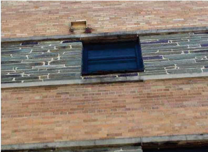
Photos 12-13. Examples of brick rotated 90 degrees at the exterior façade
