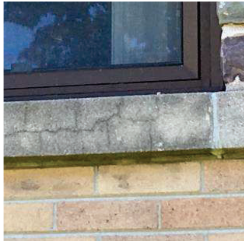
Photos 4-5. Stepped cracks in the exterior brick
