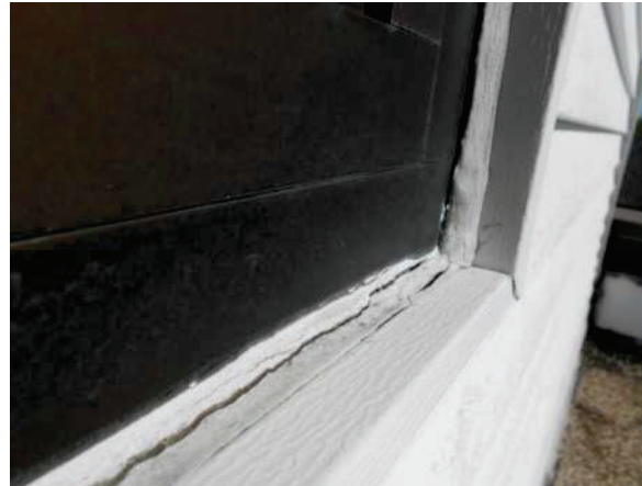
Photo 24. Example of window-to-siding trim seal
