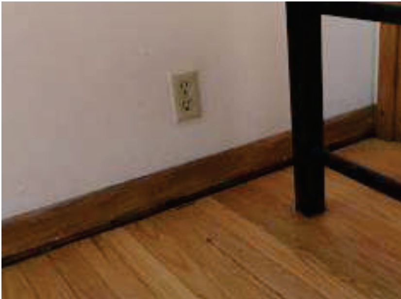
Photo 8. Settlement on the 1 st floor
