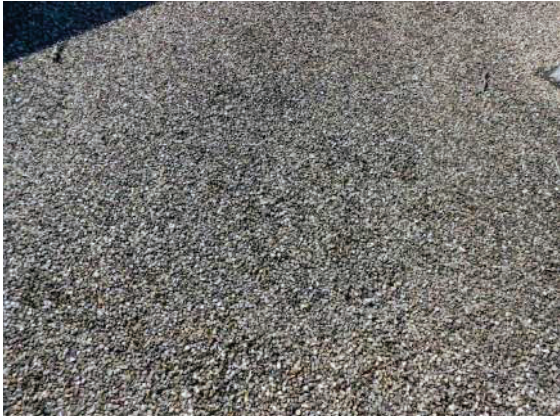
Photo 14. No blisters or soft spots in the field area
