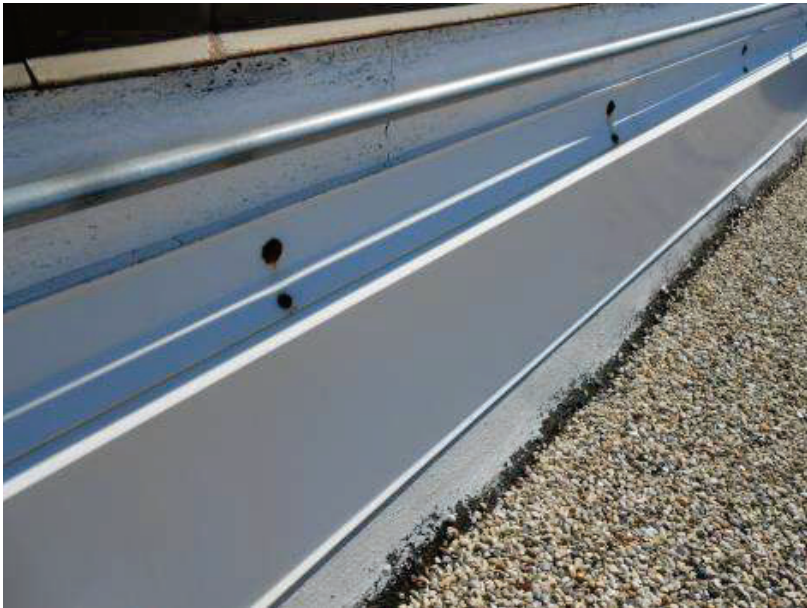
Photo 19. Example of metal counter flashing
